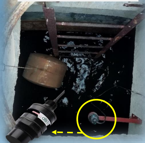
Ultrasonic Level Sensor
