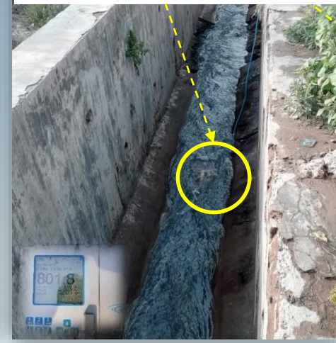
Channel Shape: Trapezoidal; Channel Dimension: 800 mm (b) x 1480 mm (B) x 2000 mm (H) x 250 mm (h)
