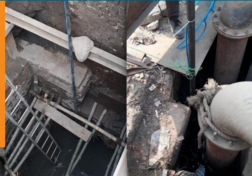
Sewer discharge monitoring in Old Trunk Sewer Lines @ Varanasi, UP
