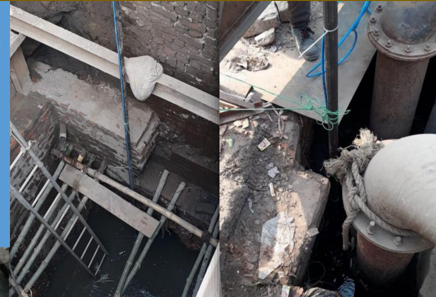
Sewer discharge monitoring in Old Trunk Sewer Lines @ Varanasi, UP
