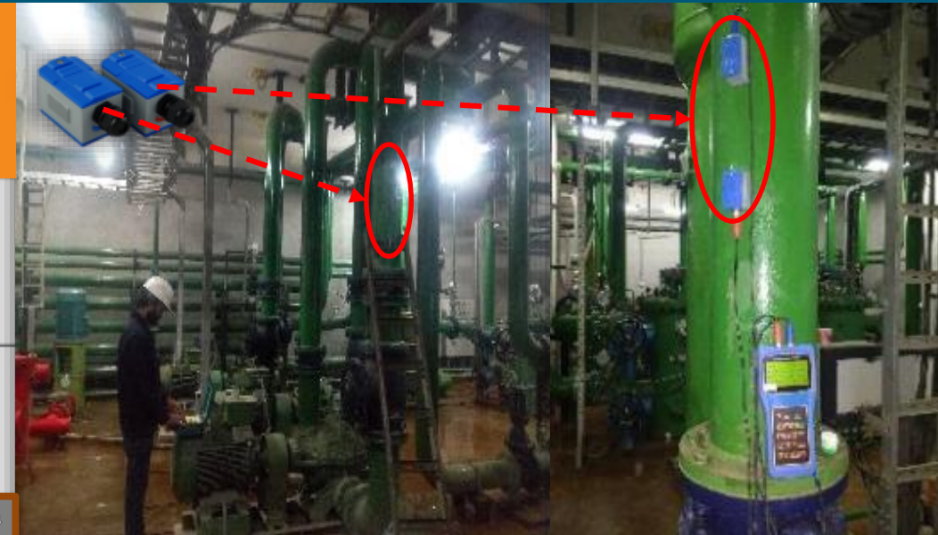
Flow survey @ (2 * 50 MW) HEP, Himachal Pradesh
